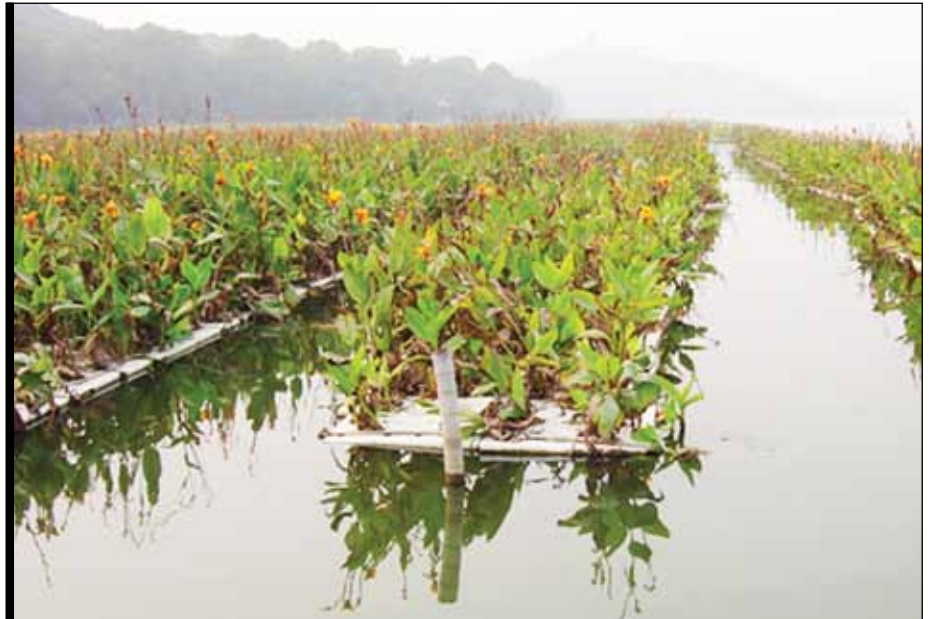
China's combined stormwater and sewerage system covers more than 10,000m 2 .
